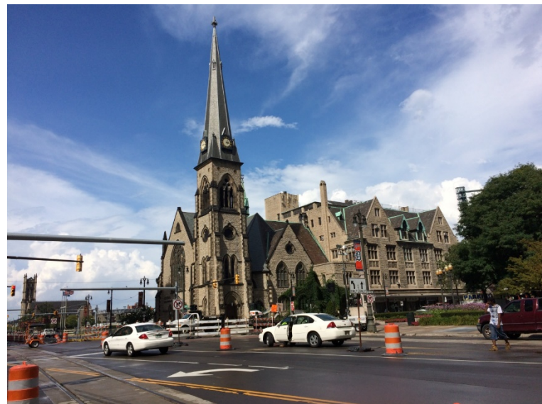
Fig.8 – Central United Methodist Church
