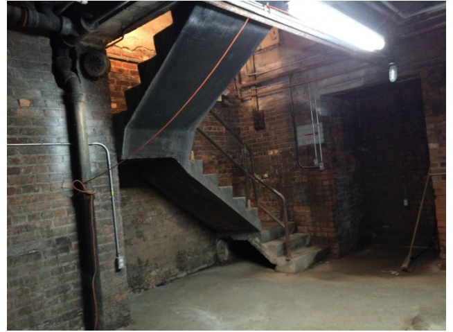
Fig.2 – Second Baptist Church, stairway for Underground Railroad
