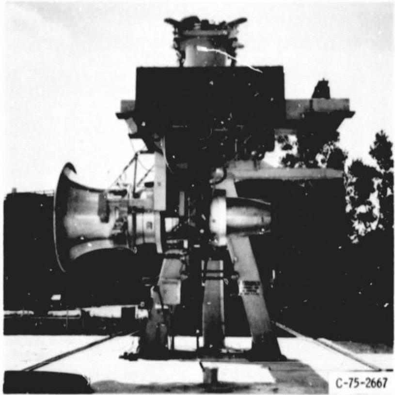
Figure 3. - YF102 turbofan engine on test stand.
