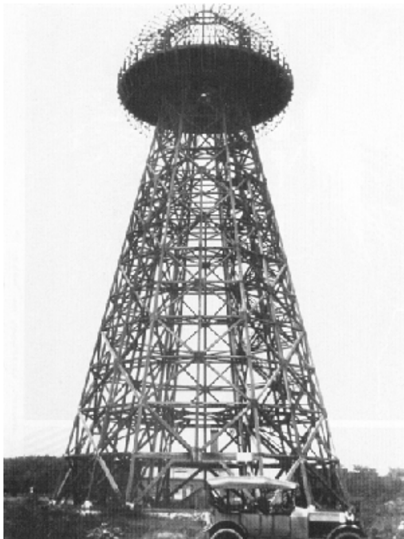
Figure 11: The skilnet of the first TESLA plant (constructed ~1901-1903) for the transmission of energy and broadcasting signals in Wardencliffe, Long Islands, New York. It was never completed.
