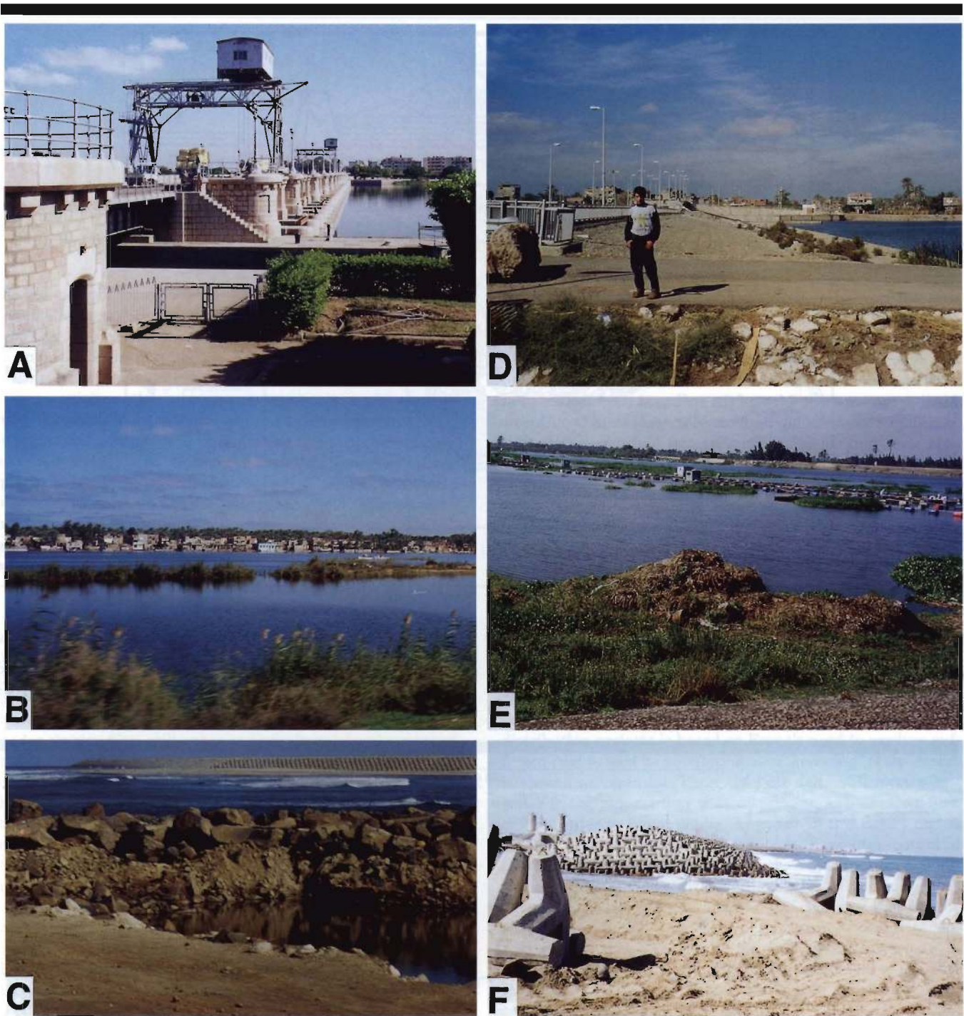
Figure 16. Photographs, taken in November 1997, showing human modification of the Rosetta and Damietta distributaries of the Nile in northern delta. (A) Edfina barrage, view towards NE (Figure 15); (B) vegetated islands forming in the Nile channel below Edfina, view towards ENE; (C) sea water entering the mouth of the Rosetta branch as shown by landward-driven waves, view towards NE; (D) Faraskur Sudd barrage, view towards NW; (E) vegetated islands and fishing huts in river channel just below Faraskur Sudd barrage, view towards W; and (F) artificial structures emplaced to protect rapidly eroding coast at the Damietta promontory, east of Ras El-Bar (in distance), view towards W.
