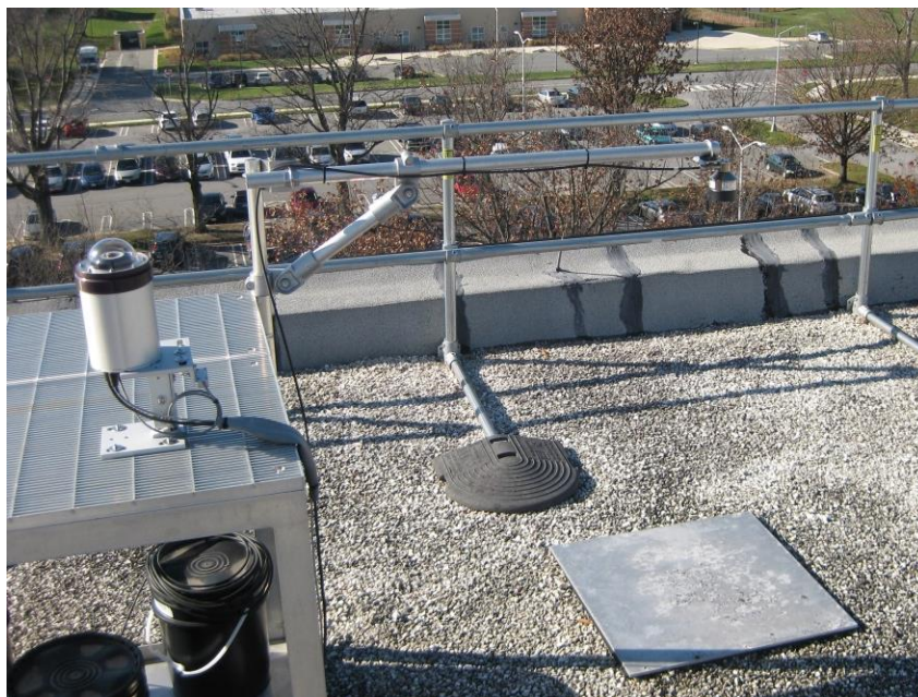
Figure 3-7 The snow sensor that measures snow depth, positioned directly above a square flat metal plate
