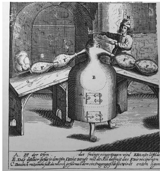
Fig. 4. One of Glauber's distillation apparatus. [26]
