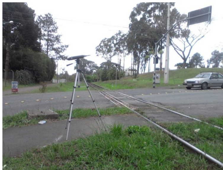
Figure 4 Urban street railroad crossing without safety barriers.
