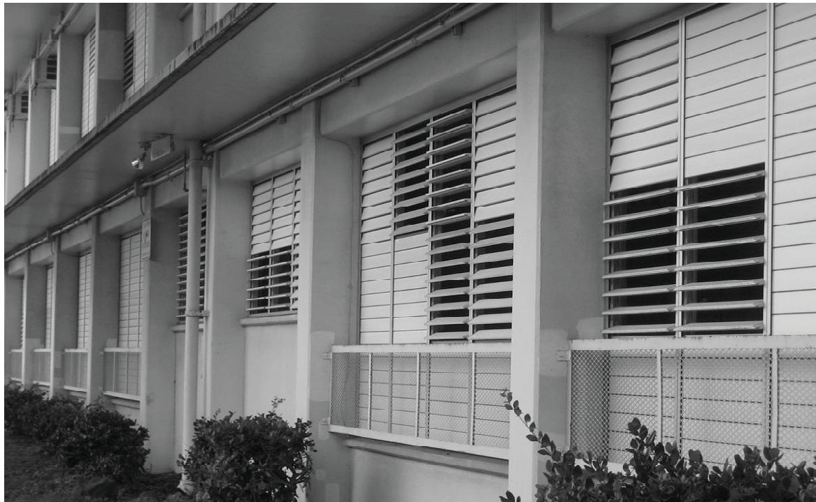
Figure 1. Photograph of jalousie windows.
