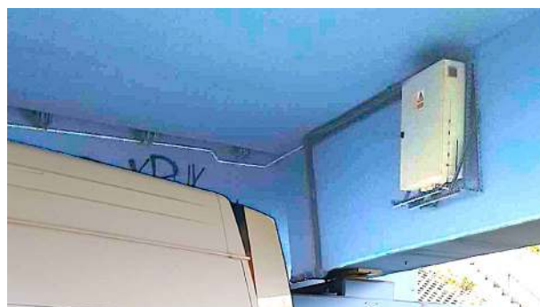
Fig. 8 Protection box under bridge
