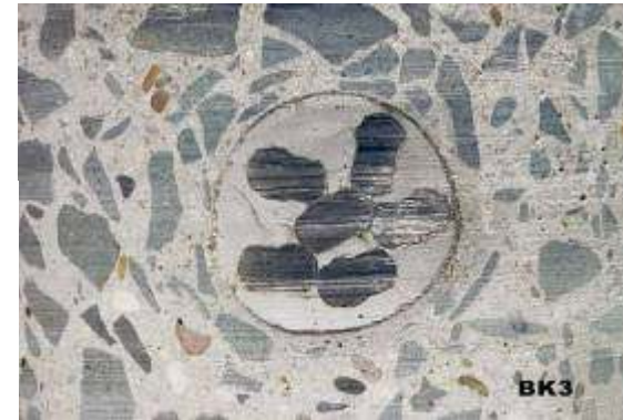
Bridge deck (transverse tendon ducts): Very good grouting condition
