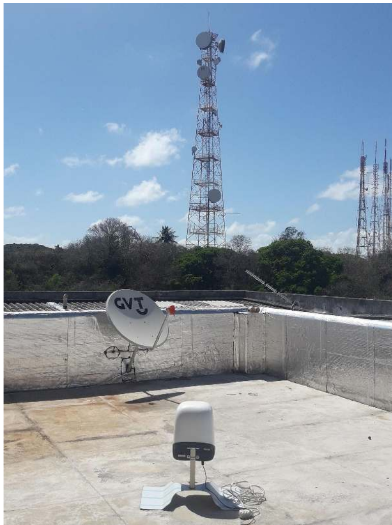
Fig. 5. Example of measurement setup and site.
