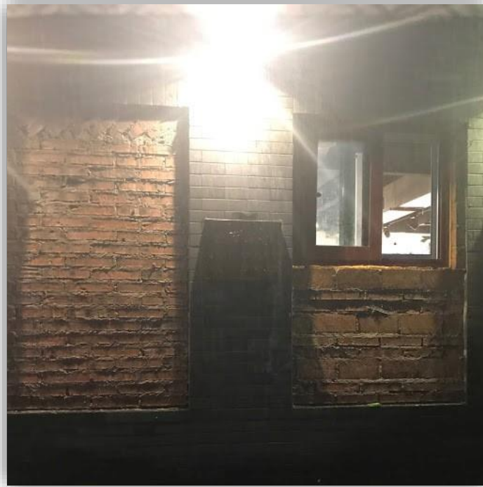
Figure 9: Bricked Up Hutong Storefront
