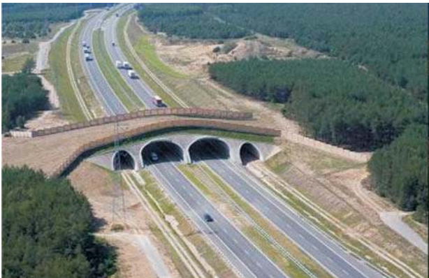
Fig. 3. Top view on the animal crossing situated on the motorway in Poland (Bednarek, Czerepak 2007)
