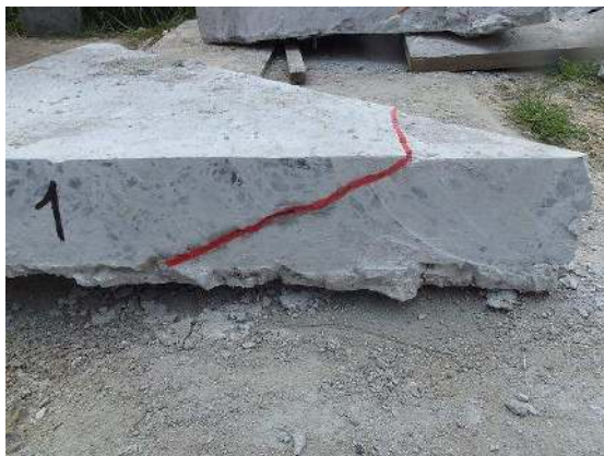
Fig. 8: Detail of shear crack – section 1
