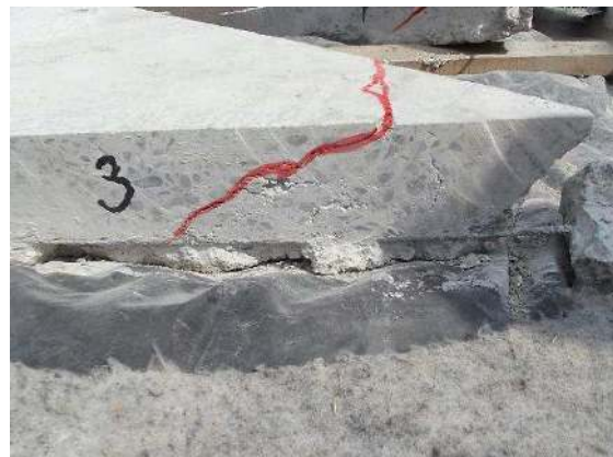
Fig. 9: Detail of shear crack – section 3.
