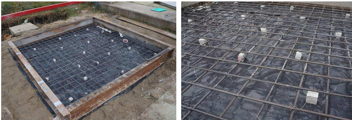
Fig. 5: The reinforcement concrete slab (left), reinforcing of the slab (right).
