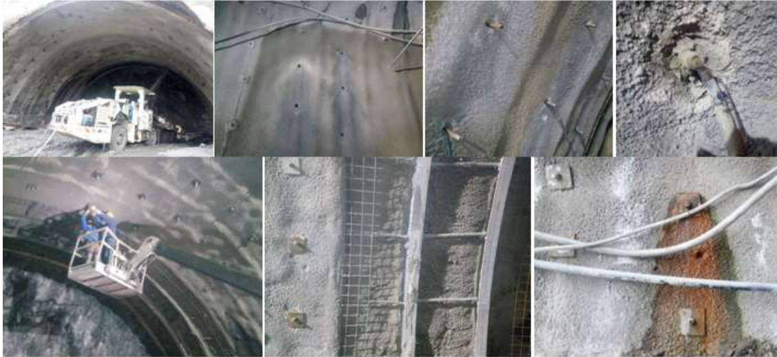
Fig. 9– Photography of tunnel Rock bolts stage
