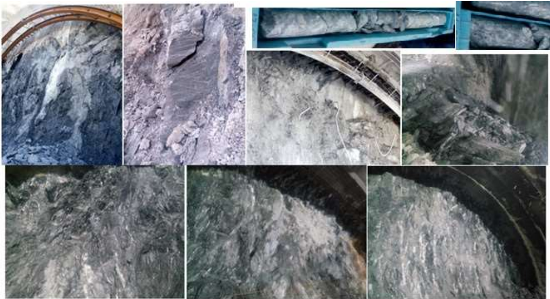
Fig. 4– Photography of tunnel alignment Geology of this study
