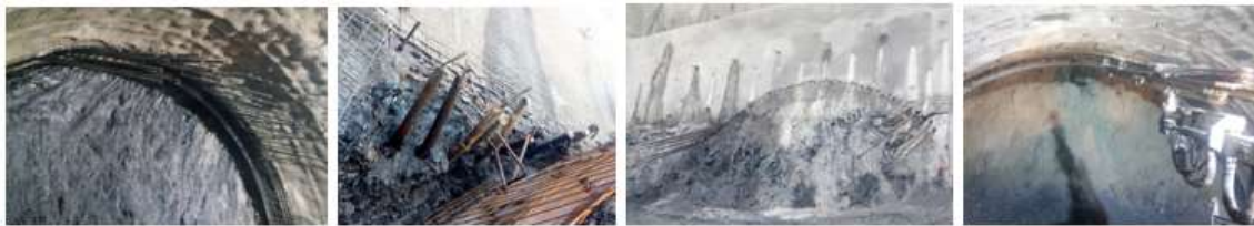
Fig. 8– Photography of tunnel pre-supporting iron bar (Umbrella) stage
