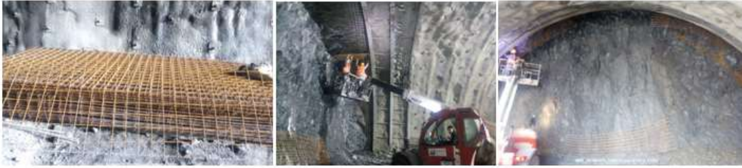
Fig. 6– Photography of tunnel Steel lattice stage
