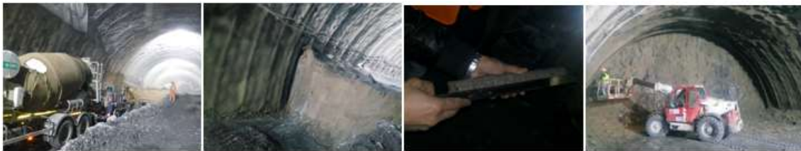
Fig. 5– Photography of tunnel shotcrete stage
