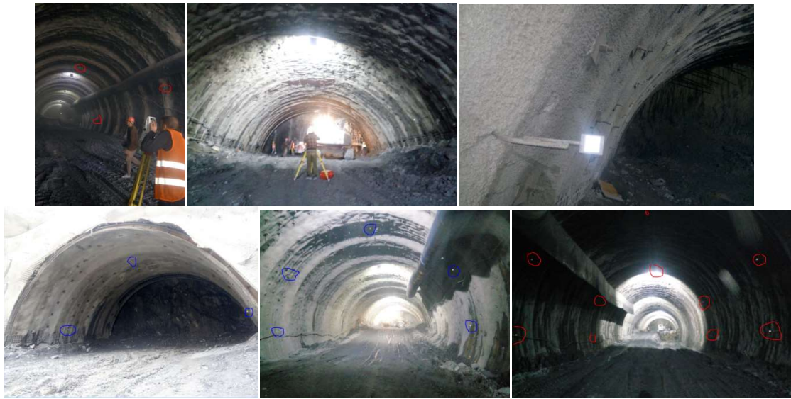
Fig. 12– Photography of the tunnel underground monitoring
