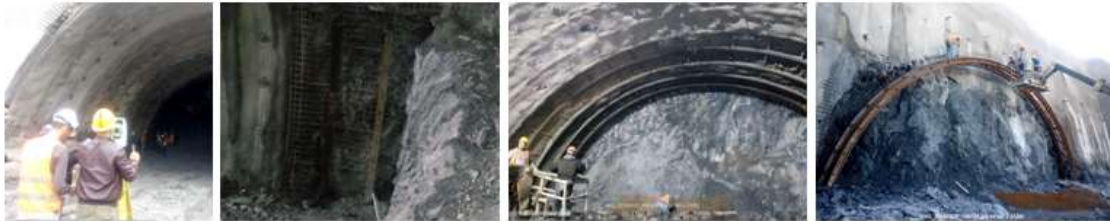
Fig. 7– Photography of tunnel Steel retaining stage
