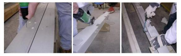
Figure 4. Notching procedure of the GFRP profiles.
