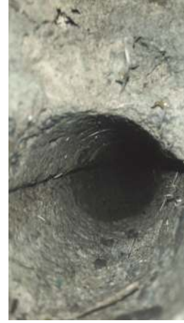
FIGURE 3: Grooved blast holes.
