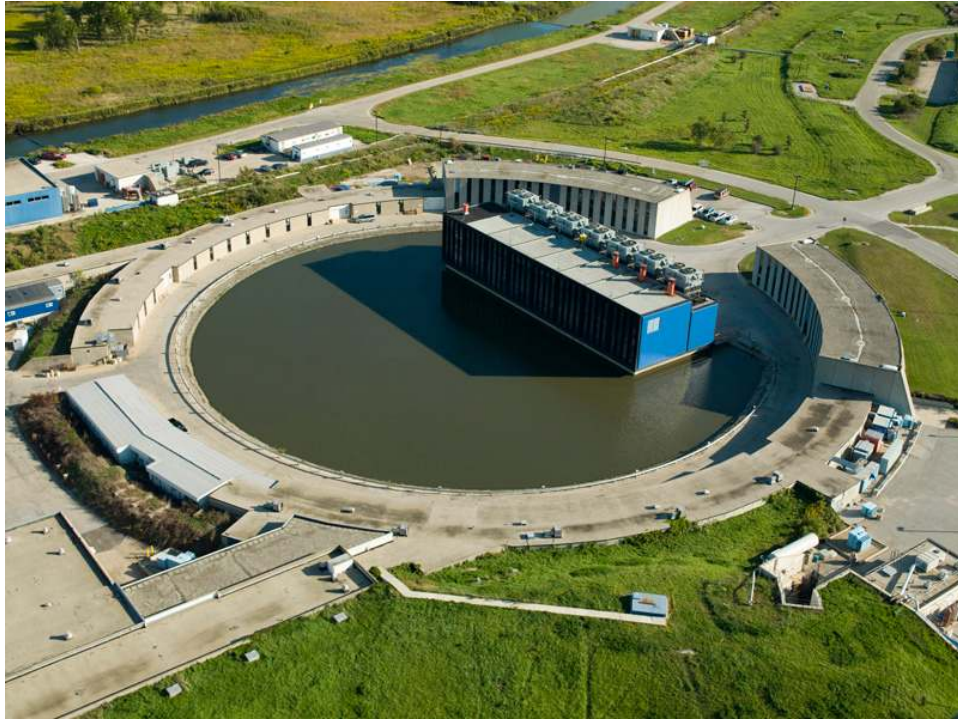
Figure 6: The Booster takes H^- ions from the Linac at 400 MeV and produces a proton beam of 8 GeV which is transferred to the Main Injector.
