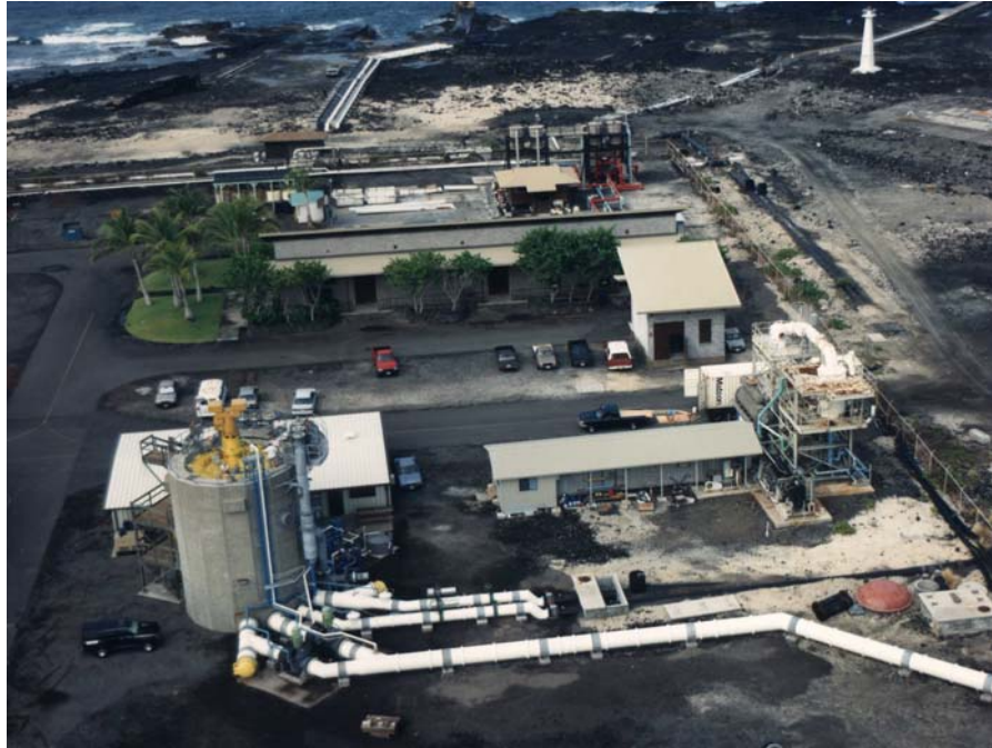
Figure 1. Photograph of 210 kW OC-OTEC Experimental Plant (1993-1998)
