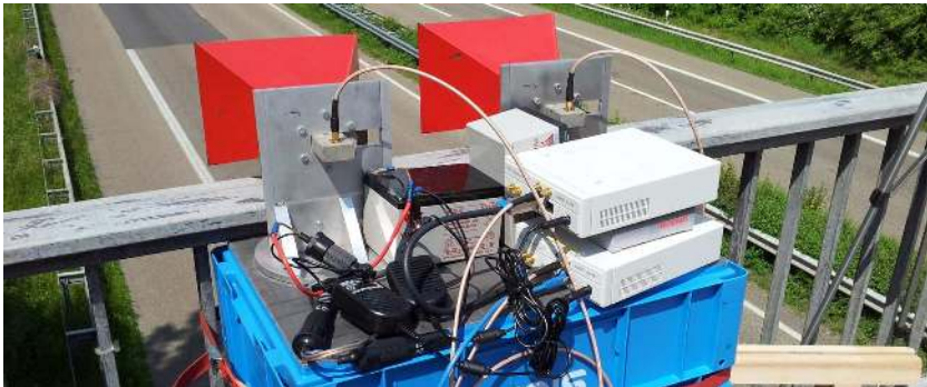
(b) Performing measurements in the field: The USRPs' power supply is a 12 V battery; DC/DC converters provide the required 6 V supply voltage.
