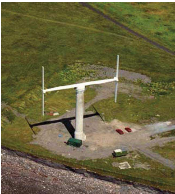
Figure 2 - 0.5MW VAWT-850 H-rotor
