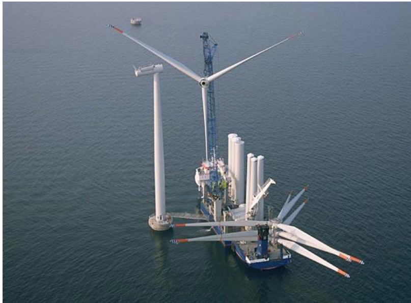
Figure 2 – Rotor blades brought to site
