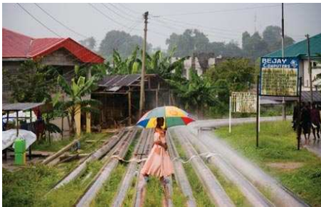
Figure 9: Oil pipelines in Okrika, near Port Harcourt
