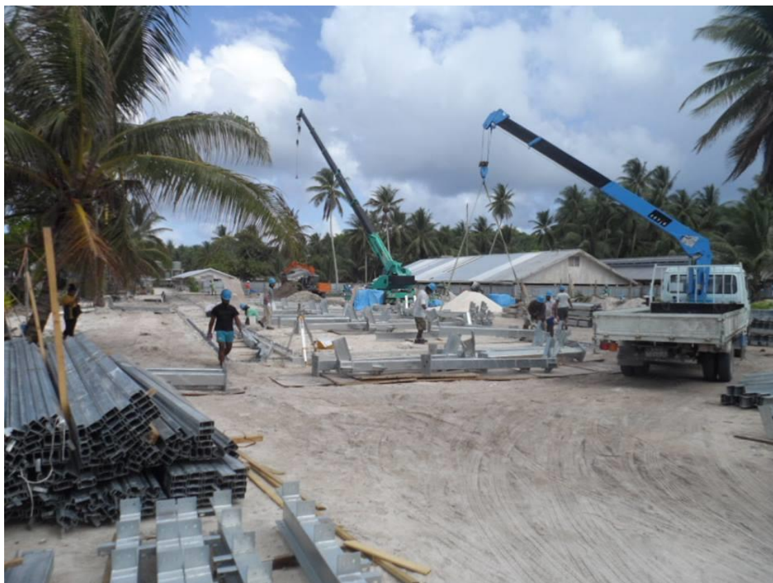
Figure 5.11: Construction of new MSS dormitories and classrooms by Japan, 2013.
