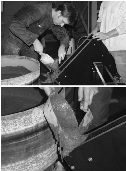
Fig. 4 Casting of the ‘U-shaped’ specimen: the mould is given an inclination to prevent free fall of the concrete along the “A”-side
