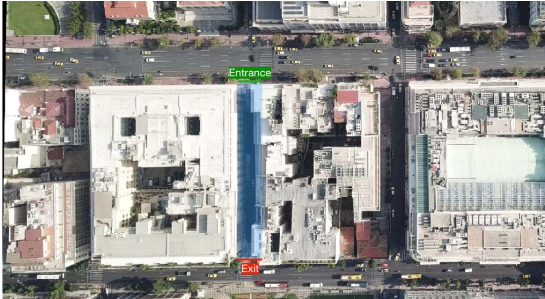
1 2 Figure 5: A minor road between two main arterial that is not visible
