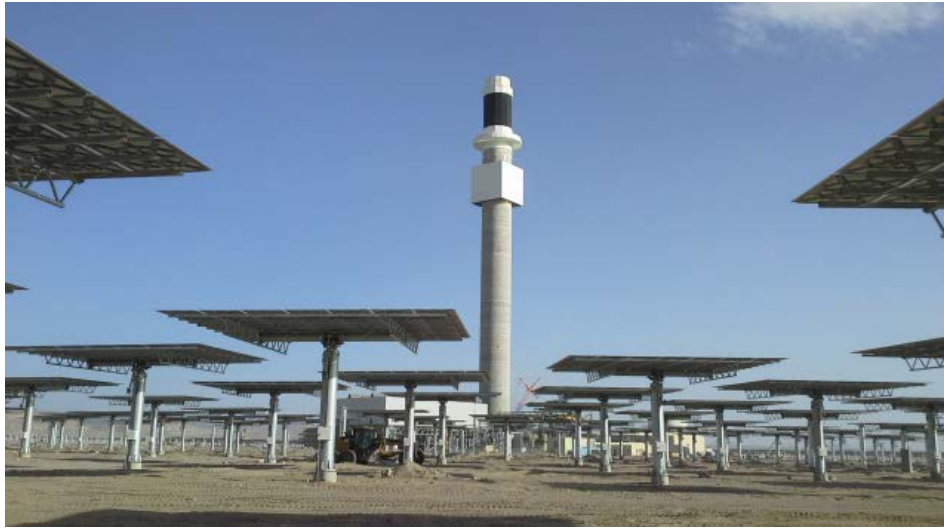
Figure 10. 110-MW e Crescent Dunes Solar Energy Project in Tonopah, Nevada, with ten hours of thermal storage
