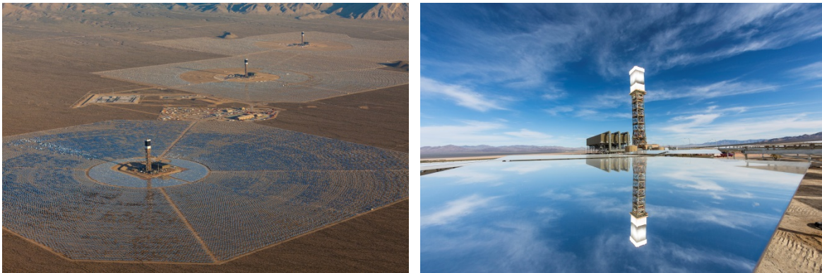
Figure 9. Ivanpah Solar Electric Generating System, which employs direct-steam heating in the receiver
