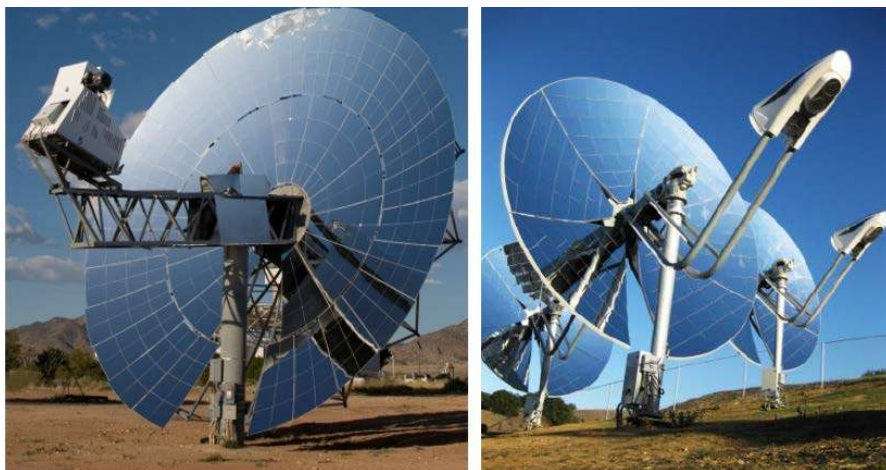
Figure 12. Two types of dish/engine systems
