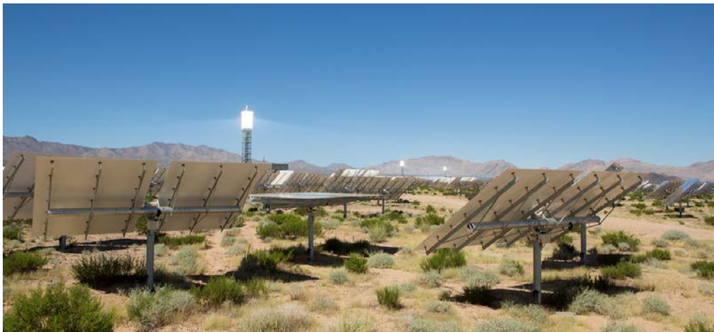
Figure 14. LH-2.2 heliostats at Ivanpah
