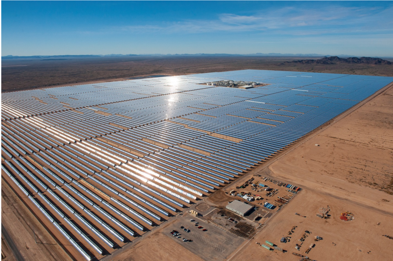
Figure 8. Solana Generating Station in Gila Bend, Arizona, which is currently the world's largest parabolic trough plant
