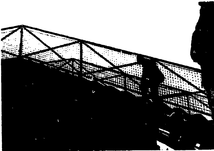
FIGURE 9. Many shapes are built from smaller ones. The reinforcing beams in a bridge illustrate how repeated patterns are used in engineering and architecture, as in nature, to form a whole out of parts.
