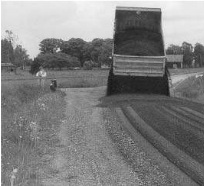
Figure 7.7 Deposition of crushed aggregate-bitumen mixture on the road.
