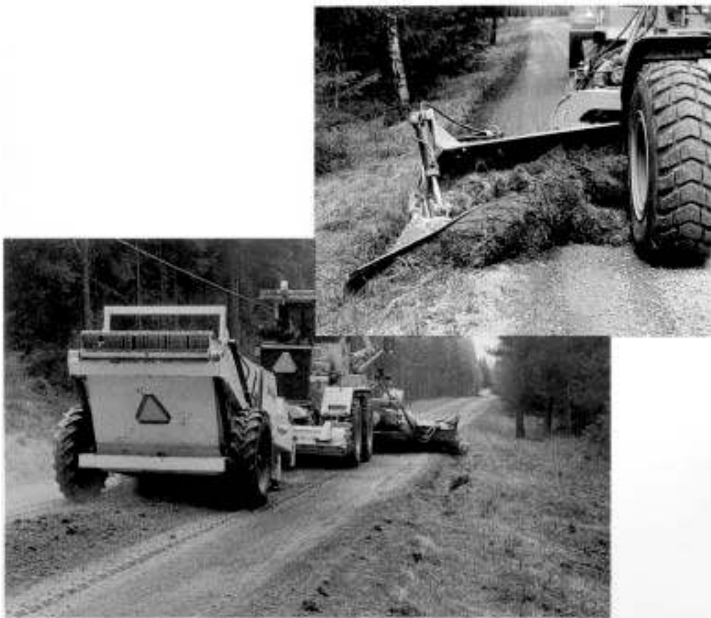
Figure 7.23 Classification with grader-drawn oversized aggregate remover; inset: edge trimmer.
