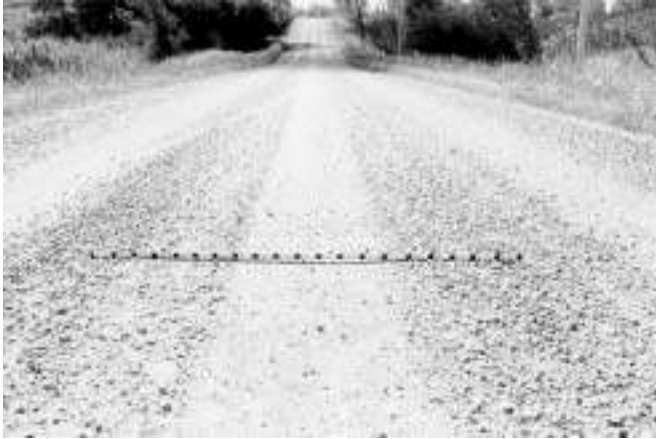
Figure 8.13 Slight rutting.
