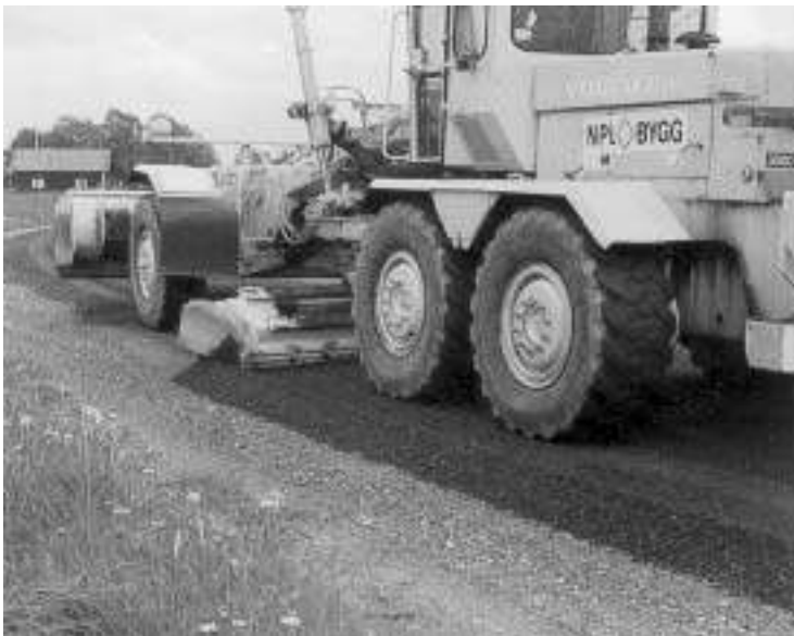
Figure 7.8 Spreading and adjustment.
