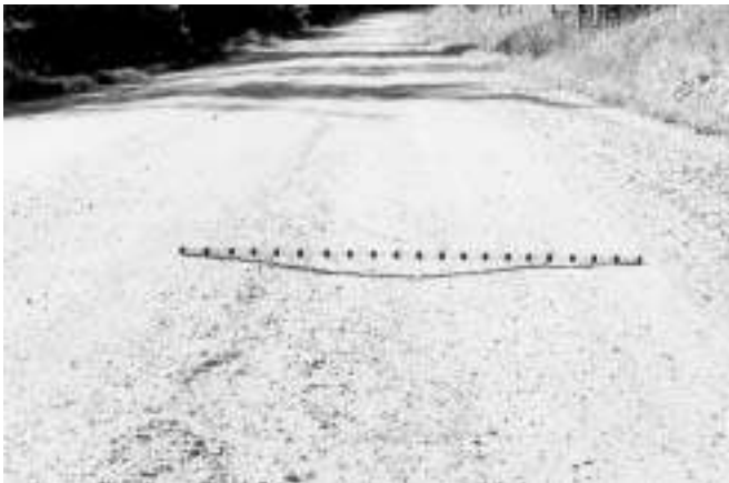
Figure 8.15 Severe rutting.
