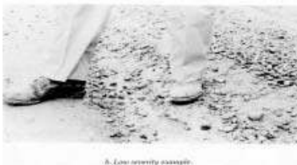
Figure 8.22 The three levels for assessment of loose aggregate (Eaton and Beaucham, 1992).
