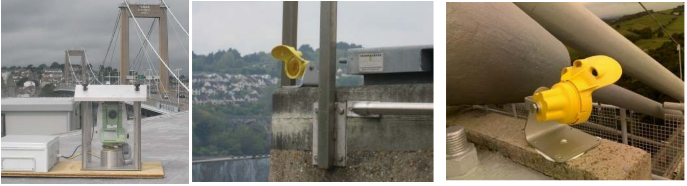
Figure 5: RTS unit on control room roof (left) and reflectors on Plymouth side tower (middle) and Saltash Tower (right).
