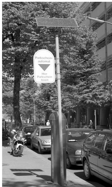
Figure 3: Photovoltaic module that supplies electricity to a parking ticket machine in Berlin, Germany. Photo: M. Brogren.
