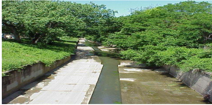
Figure 7-3. Section of concrete channel in South Fork of Beargrass Creek
