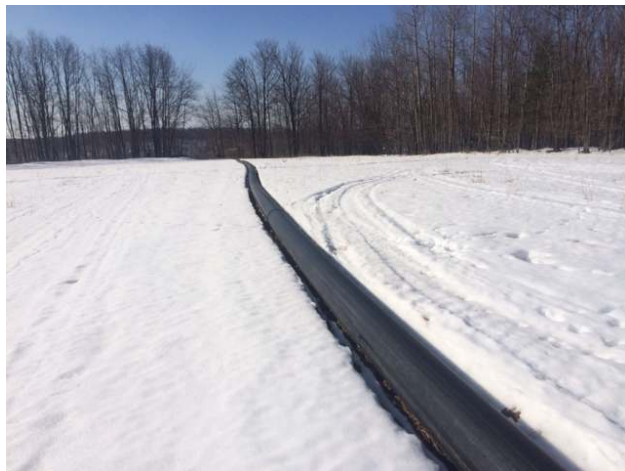
Figure 5: Water transportation through temporary piping
