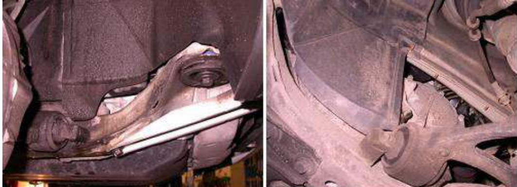
Figure 11 Gap between wheel arch liner and the sub frame on a XC90
