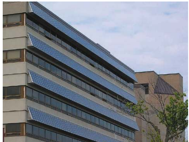
Fig. 1 Queen's University's first 20 kW solar PV array (photo: Anton Driesse)
