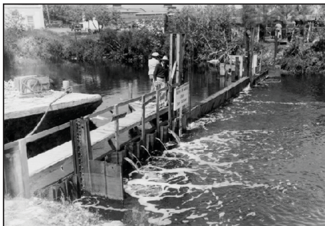
Figure 12. First water control structure on the Miami Canal installed in December 1939. This structure leaked considerably and also was opened to allow barges to pass. Photograph from the files of the U.S. Geological Survey.
