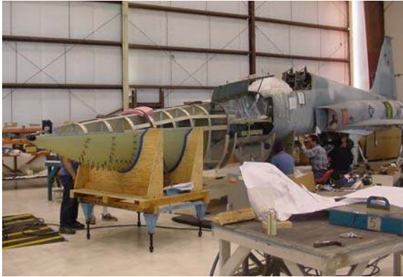
Figure 20. Installation of new nose and fairings are required as part of the SSBD modification.
