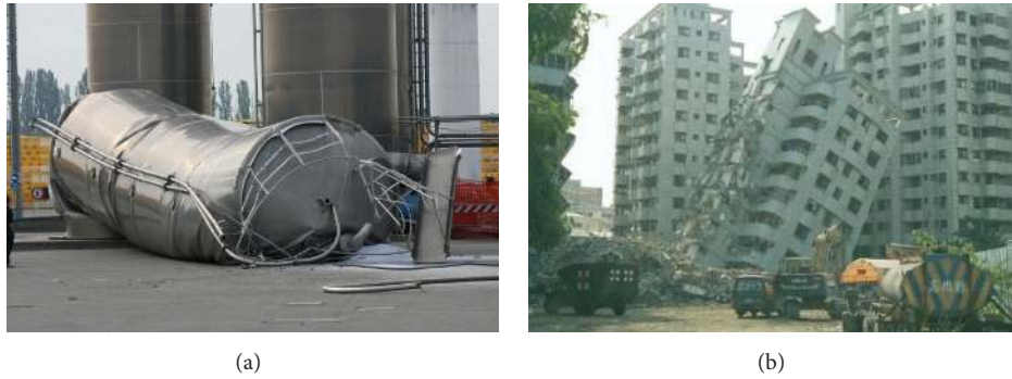
FIGURE 1: Catastrophic collapses due to earthquakes.
