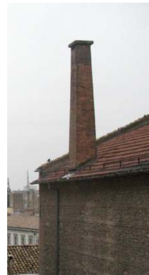
FIGURE 3: An old masonry chimney.
