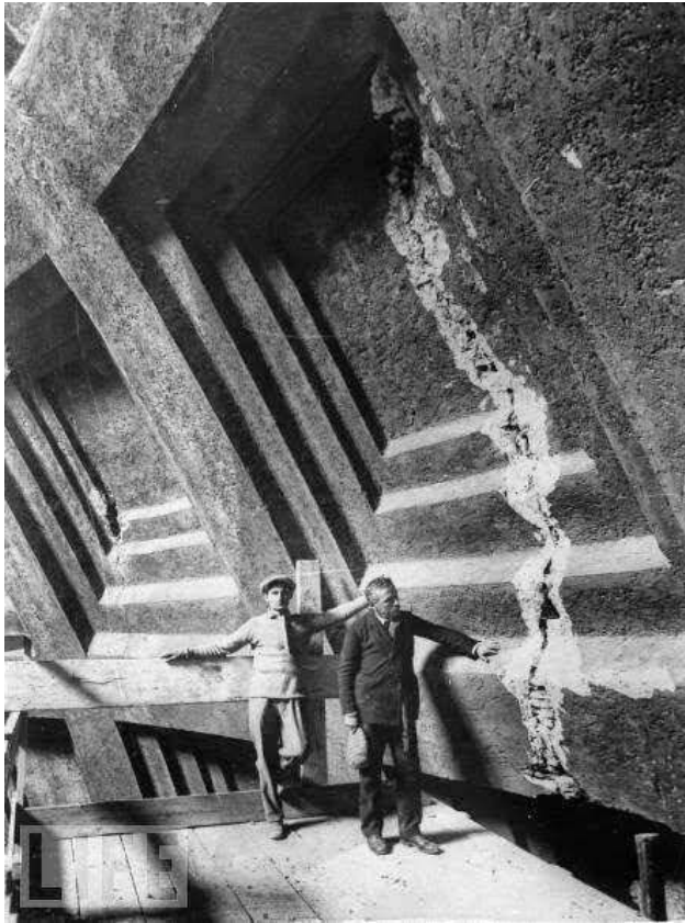
Figure 12: A vertical creep in Pantheon dome during restoration works in 1925
