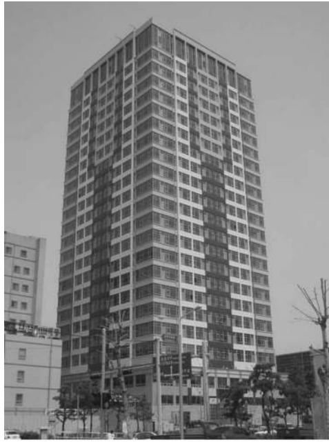
(a) Overall view
