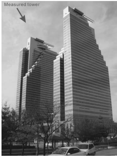
(a) Overall view
