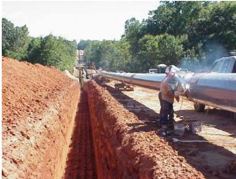
FIGURE 3.3-10 Welding Pipe (Source: Photos courtesy of U.S. Pipeline, Inc. Reproduced with permission.)
