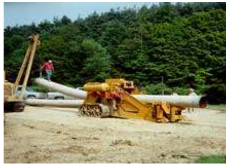
FIGURE 3.3-11 Pipe Bending Machine
