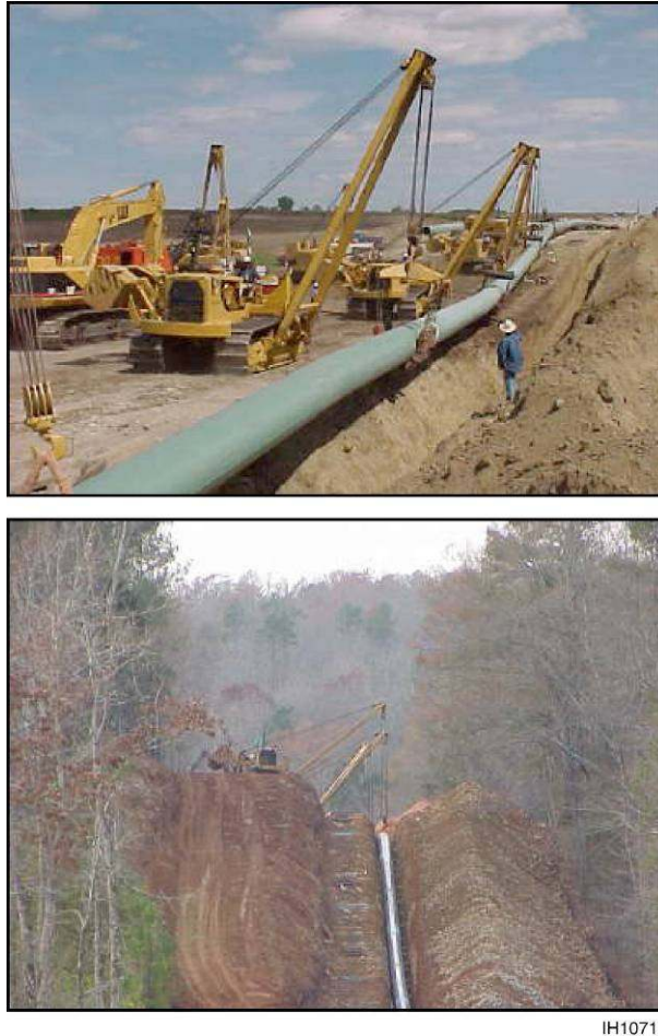
FIGURE 3.3-13 Lowering Pipe into Trench (Source: Photos courtesy of U.S. Pipeline, Inc. Reproduced with permission.)
