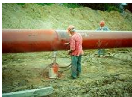
FIGURE 3.3-12 Applying Coating to Pipeline
