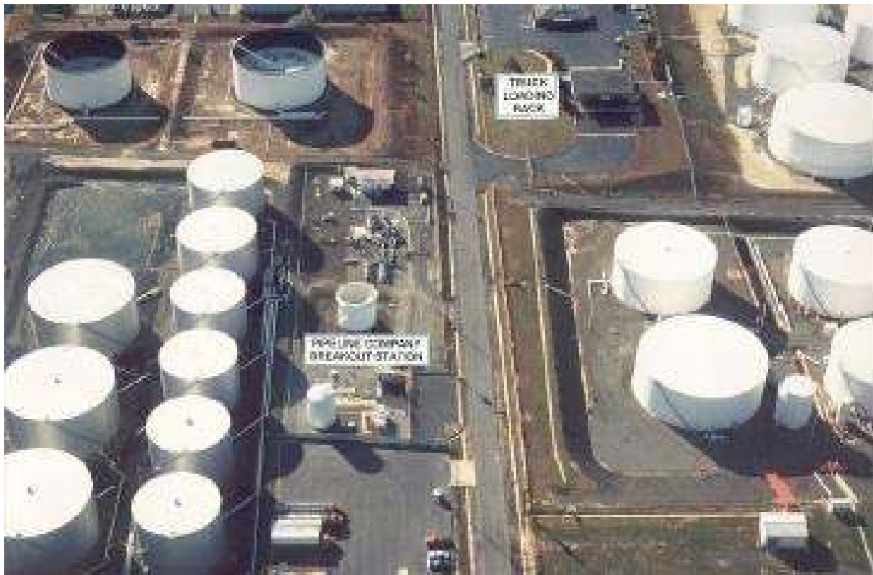
FIGURE 3.3-27 Typical Pipeline Breakout Station (Terminus) at a Petroleum Terminal (Source: V. Yarborough, Argonne staff)
