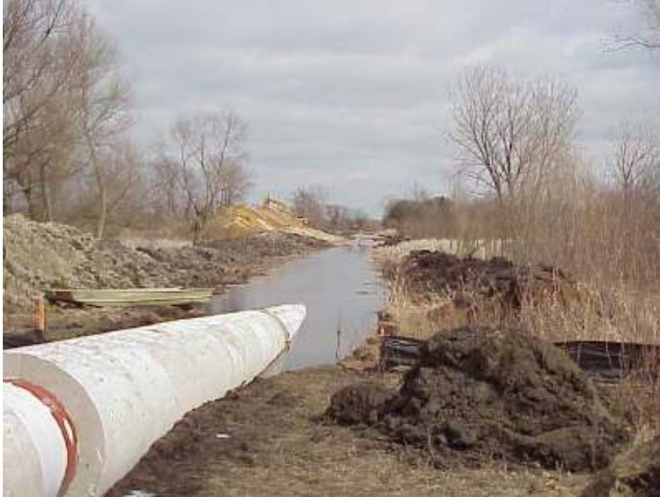
FIGURE 3.3-25 Concrete-Coated Pipe in a Wetland (Source: Photo courtesy of U.S. Pipeline, Inc. Reproduced with permission.)
