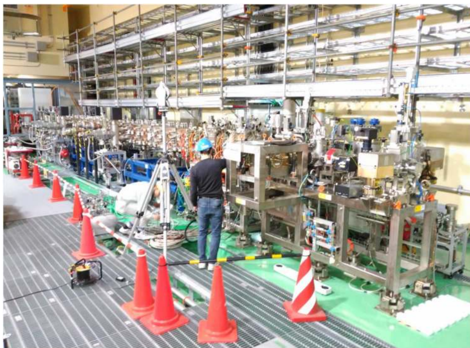
Figure 14. LIPAc accelerator during its alignment in Rokkasho Fusion Institute at the time of the drafting of this article. From left to right one can appreciate the injector, the RFQ, the MEBT and the diagnostics plate.
