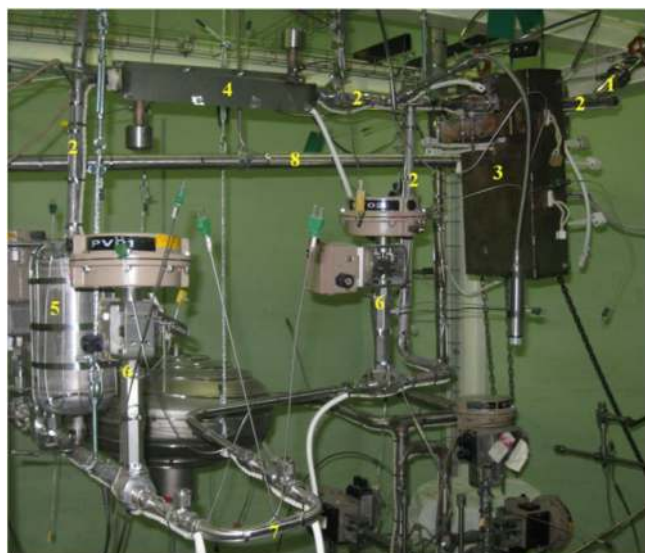
Figure 12. View of Li loop LiFus 6: (1) regulating valve (connected to the main loop); (2) purification loop pipe; (3) resistivity meter; (4) air cooler upstream of the cold trap; (5) cold trap; (6) pneumatic valves to permit/exclude Li circulation in the sampling tube; (7) sampling 'U' tube; (8) pipeline of the main LiFus 6 loop.
