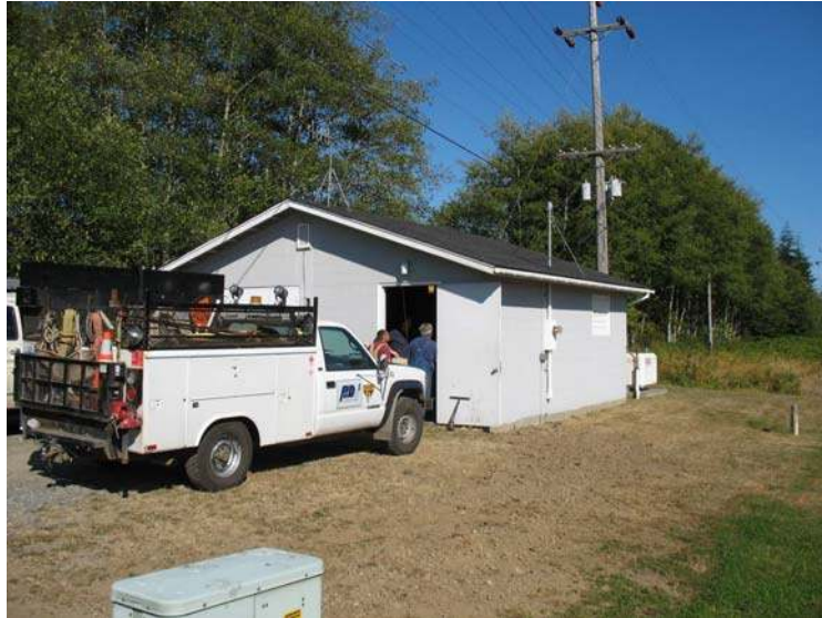
Figure 5.3. The Sekiu Pump Station Located Across the Street from Clallam PUD Facilities
