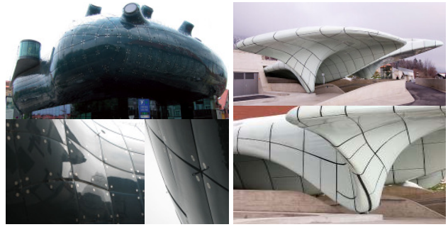
Figure 2: Projects involving double-curved panels where a separate mold has been built for each panel. These examples illustrate the importance of the curve network and the challenges in producing architectural freeform structures. (Left: Peter Cook and Colin Fournier, Kunsthhaus, Graz. Right: Zaha Hadid Architects, Hungerburgbahn, Innsbruck.)
