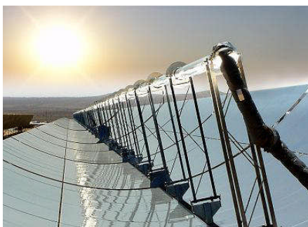
Figure 8. Parabolic mirror facets.
