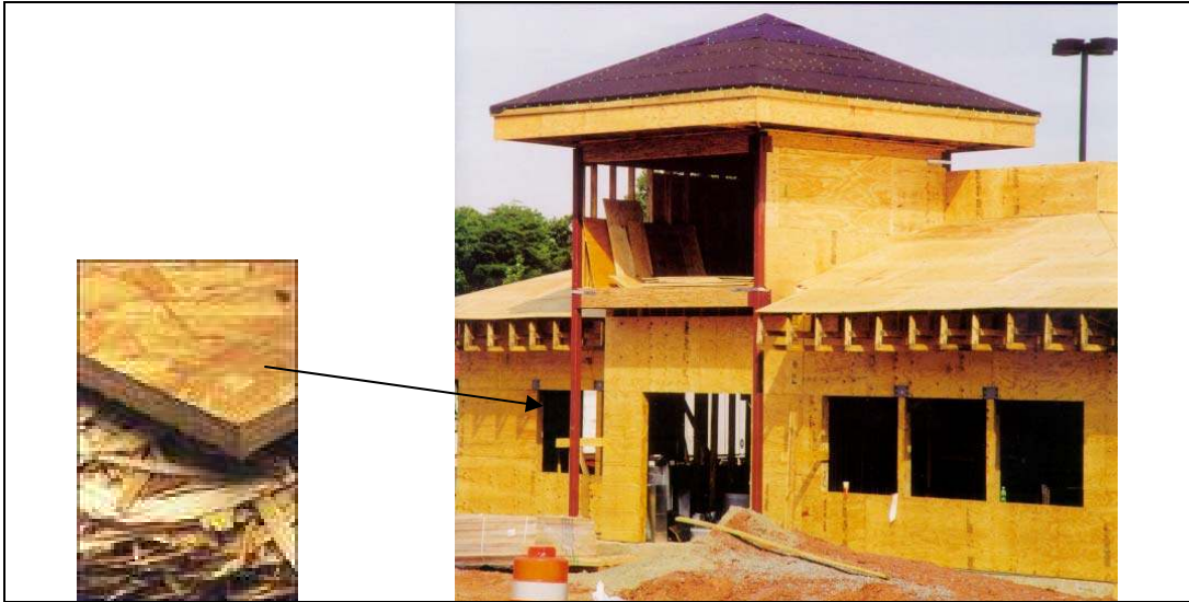
Figure 2.5. Illustration of OSB wood strands, panels and uses in construction.
