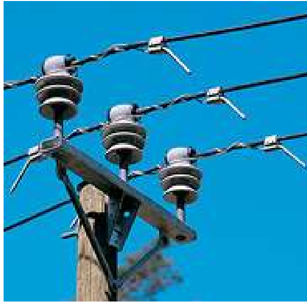
Fig. 2.2 Construction of a typical PAS line – Suspension pole with pin insulators and lightning protection using APDs implemented with arcing horns [13]
