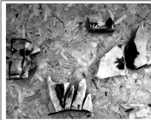
Figure 17 – Evidence of internal partial discharges occurring within the failed transformer porcelain bushing
