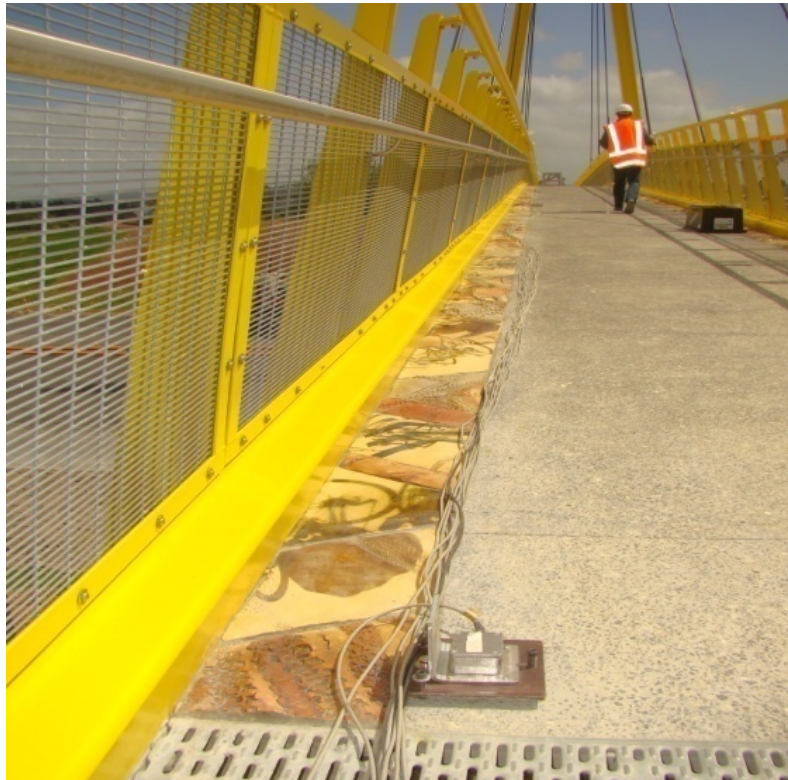
Figure 5. Accelerometers (in the center) and shakers (at the back) placed on the bridge.
