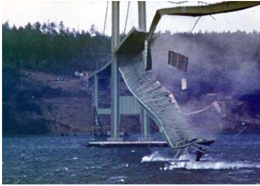
Fig. 1 The collapse of the Tacoma Narrows Bridge on 7 November 1940.
